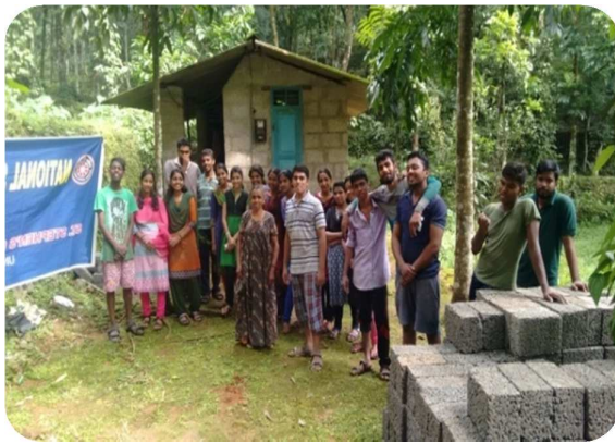
Sanitary Block Construction to a lonely lady,
